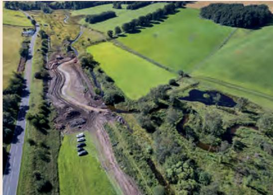
Figure A1.9 Eddleston Water re-meandering (stage 2) during construction. Earlier re-meandering undertaken as part of stage 1 is also visible (courtesy Tweed Forum)
