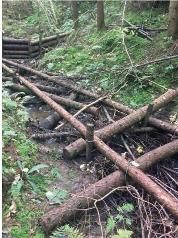
Figure 10.12 Interlocking/lattice jam leaky barriers (courtesy West Cumbria Rivers Trust)
