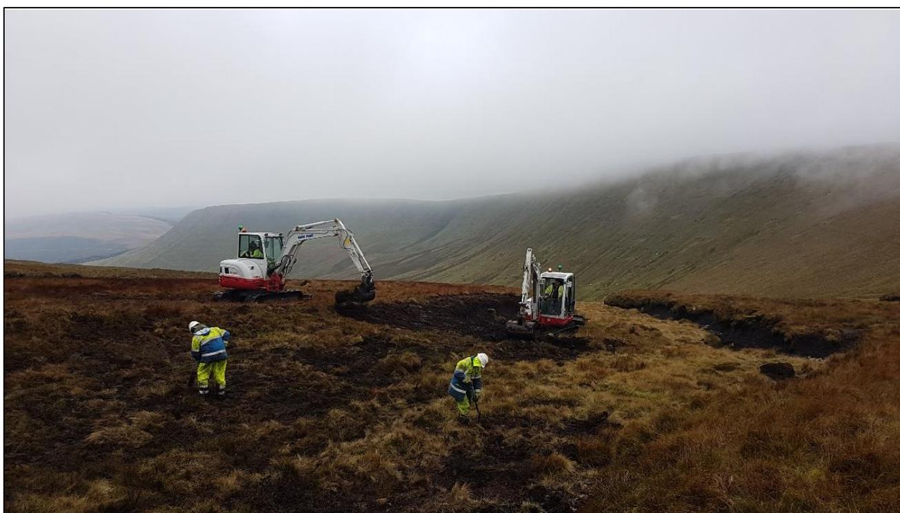
**Figure 2.4 | Hagg re-profiling at a site in the Brecon Beacons.** Two diggers work on the hagg – the one on the top of the hagg is laying down the turf, teasing it out and pressing it down firmly. The digger at the bottom of the hagg has just re-profiled the peat. There are also two workers with forks filling in any remaining gaps in the vegetation. Few borrow pits were used and any that were created were small and easily covered up by teasing out the vegetation (Photo: Rachel Harvey, SNPA).
