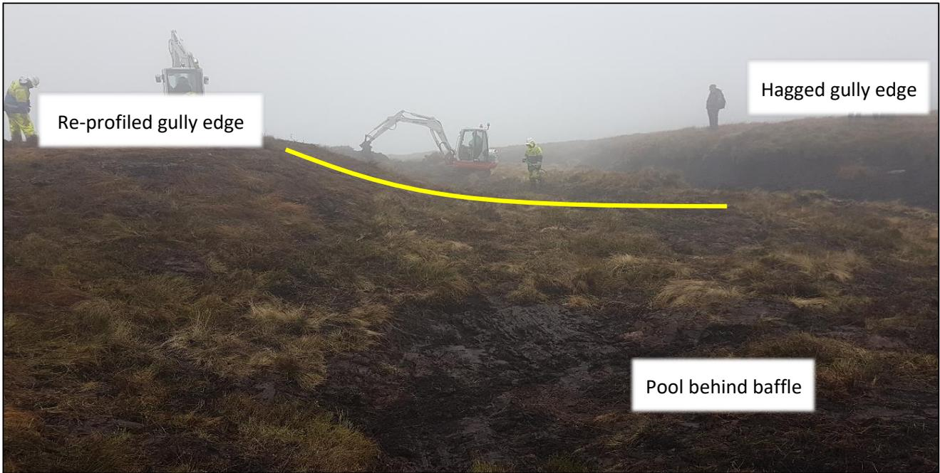
**Figure 3.7 | A peat baffle in a gully.** An example of a peat baffle in the Brecon Beacons (the baffle is highlighted by the yellow line). This baffle is approximately four metres long and stretches across more than half the width of the gully. A small pool (less than ten centimetres deep) has been created behind the baffle to facilitate colonisation of peat-forming vegetation such as *Sphagnum* moss.
